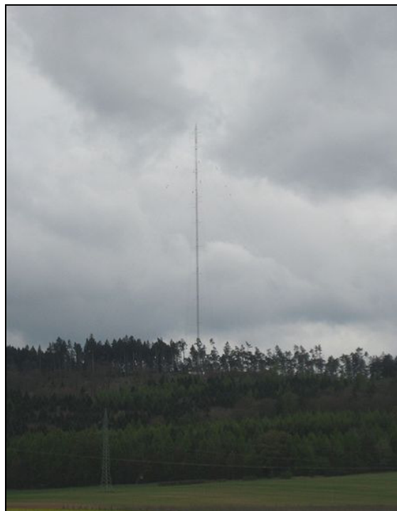
Figure 4-33 Wind measurement mast
